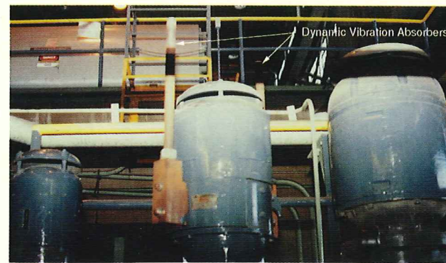
Figure 7. Emergency DC lube oil pump motor with two DVAs attached.
